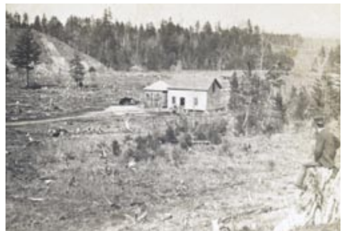
Figure 4. View of clear cut area, Champlain Spring, Highgate, Vermont, late 1800s. In the background are landslides on a steep, cleared slope. Field work suggests failures are in silty, fine sand, glacial lake deposits of the Champlain lowland. These shallow planar slides were likely catalyzed by loss of effective root strength after clear-cutting of the slope (see Fig. 3). In the middle ground are many stumps and much slash, the remains of cutting second-growth timber. There is a spring house at the center of the image. Note the tremendous size of the stump on which the man is sitting; it is likely all that remains of the old growth, pre-settlement forest that once covered Vermont lowlands like this. Image property of University of Vermont, Special Collections, Bailey Howe Library (LS03668).
