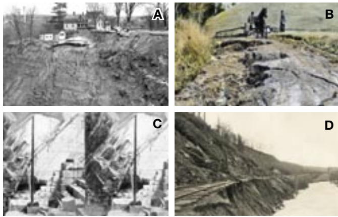
Figure 1. Images from the Landscape Change Program archive depicting landscape features, changes, and processes of interest to geoscientists. (A) Photograph of a large landslide that occurred in Burlington, Vermont, in December 1955. Slide is in glacial-lacustrine and glacial-marine silt and clay and was triggered by a leaking drain pipe. LS01781, image property of Bailey Howe Library, Special Collections, University of Vermont. (B) Hand-colored lanternslide of a horse and buggy on a washed-out road in St. Johnsbury, Vermont, 1914. LS06469, image property of Vermont State Archives. (C) Quarrying marble, West Rutland, Vermont. Stereoview shows structure of rock in high wall of quarry. LS05073, image property of Bailey Howe Library, Special Collections, University of Vermont. (D) Photograph showing erosion undercutting railroad tracks in Barton, Vermont, after 1927 flood of record. Slopes above tracks are unvegetated and failing. LS02477, image property of Old Stone House Museum.
