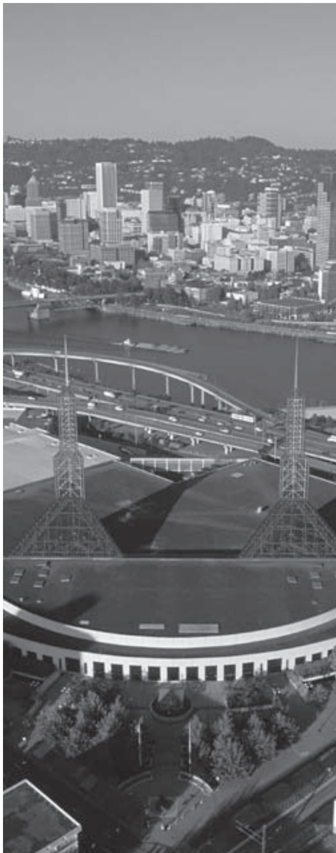
Oregon Convention Center. Photo by Bruce Forster courtesy the Portland Oregon Visitors Association.
