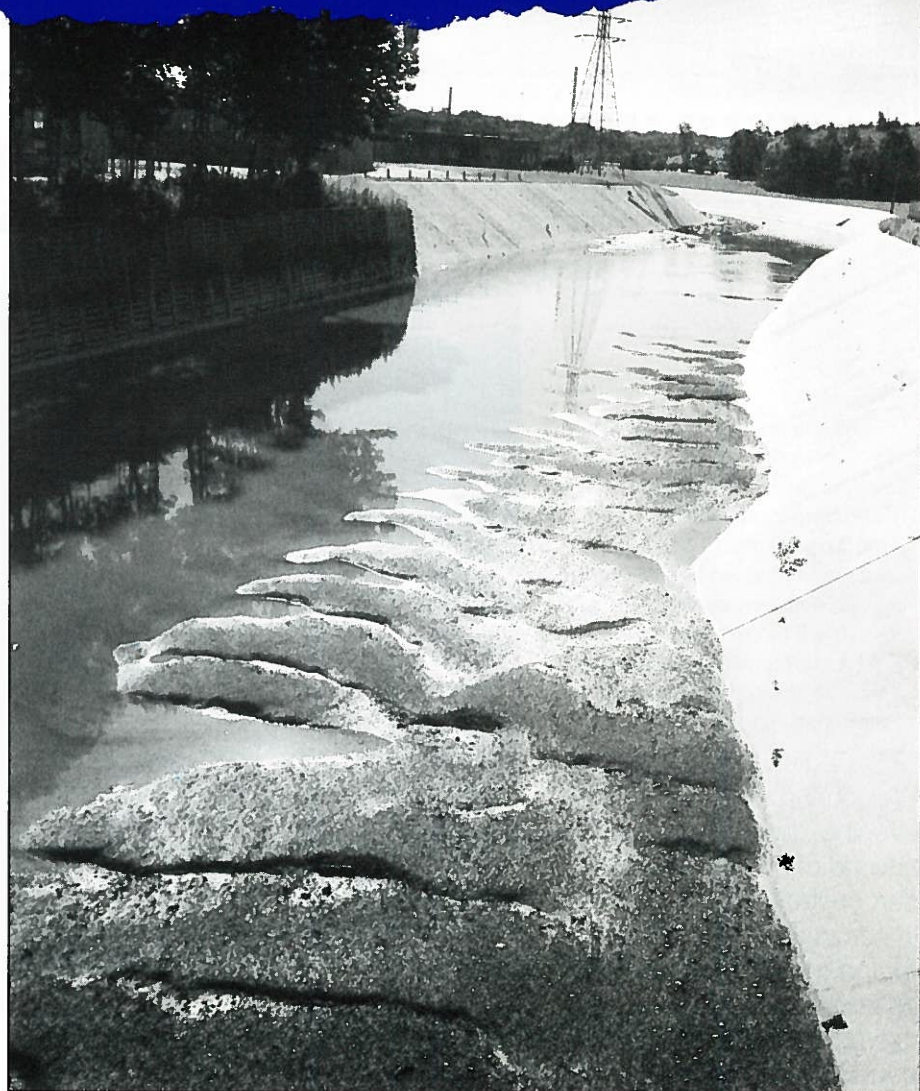
Sand waves at bridge over Mill Creek, Cincinnati, Ohio. Photo by Paul Potter, University of Cincinnati.
