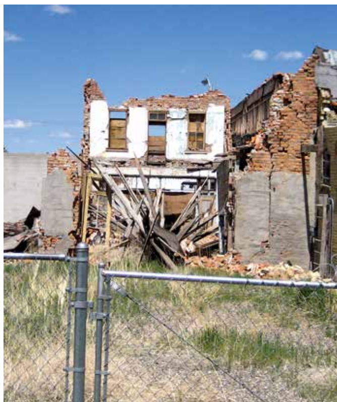
Figure 14. Front (left) and back (right) of an unreinforced masonry (URM) building damaged in the 21 Feb. 2008 Wells earthquake in Nevada, USA.
