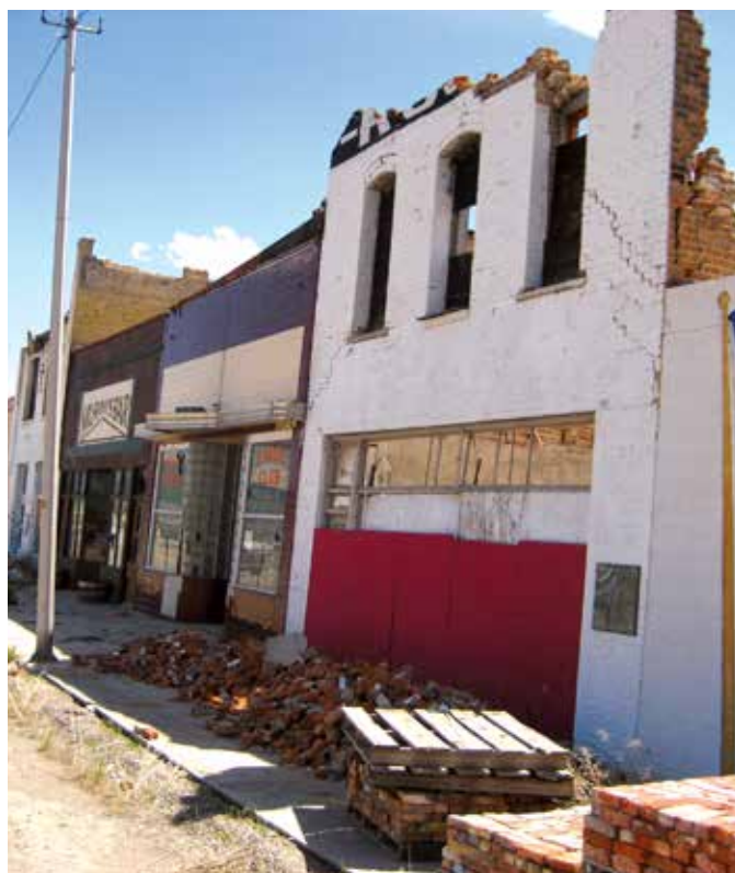
Figure 14. Front (left) and back (right) of an unreinforced masonry (URM) building damaged in the 21 Feb. 2008 Wells earthquake in Nevada, USA.
