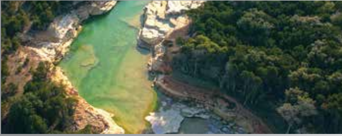
Aerial overview of the Canyon Lake spillway of south-central Texas. Photo by Larry Walther.
