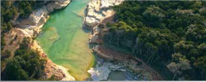
Aerial overview of the Canyon Lake spillway of south-central Texas. Photo by Larry Walther.
