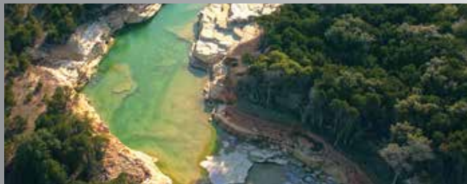
Aerial overview of the Canyon Lake spillway of south-central Texas. Photo by Larry Walther.
