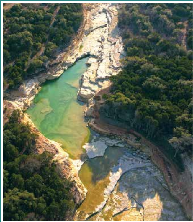
Aerial overview of the Canyon Lake spillway of south-central Texas. Photo by Larry Walther.
