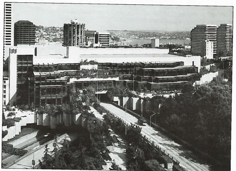
Washington State Convention and Trade Center. Photo courtesy of Seattle-King County Convention and Visitors Bureau.
