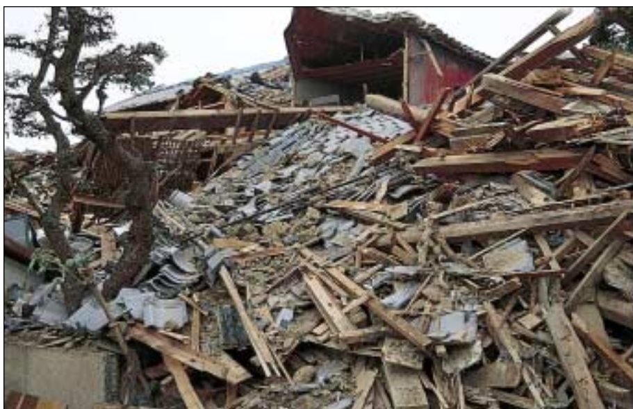
Figure 6. Collapsed Japanese wood-frame home. (Photograph by Carol S. Prentice, U.S. Geological Survey.)
