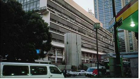
**Figure 8.** Collapsed sixth story in eight-story Kobe City Hall Annex, a reinforced-concrete building built in the 1960s. Behind it is the 16-story New City Hall, a 1980s steel-frame building that was not damaged and remained functional after the earthquake. (Photograph by Christopher Rojahn, Applied Technology Council.)
