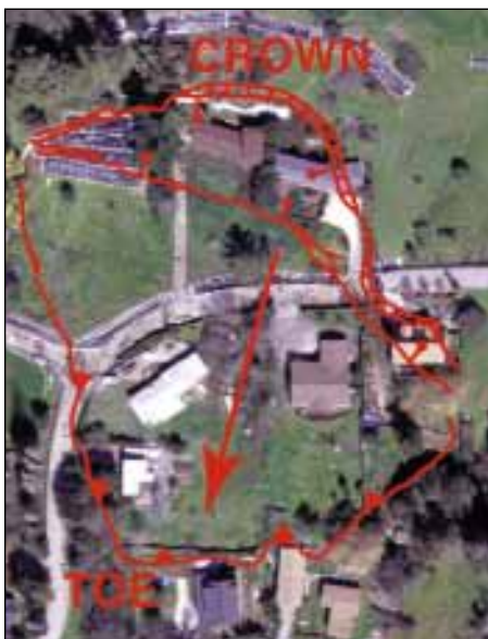
Figure 11. Ancient landslide reactivated in early 1998, at Scenic Drive, La Honda. Head scarp has deformed house in upper right. After Jayko et al. (1998).
