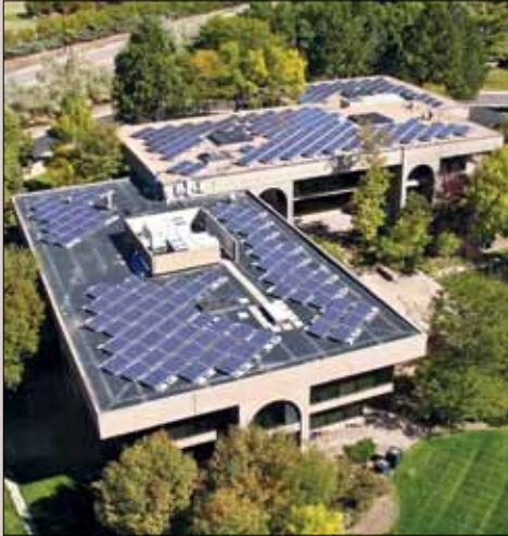
Aerial photo of the GSA headquarters solar array.
