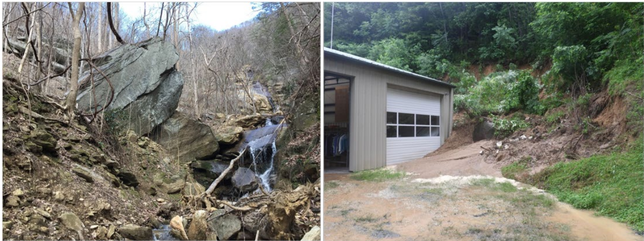
Figure 3-8. Left: View looking upslope (north) along the path of the debris flow (embankment failure) that damaged a Village of Chimney Rock park. 2019 NCGS photo. Location A – Figure 3-9. Right: Damage to the Chimney Rock Volunteer Fire Department (CRVFD) by a May 30, 2018 debris slide (cut slope failure) triggered by subtropical depression Alberto. View looking northwest. 2018/05/30 CRVFD photo. Location B – Figure 3-9.
