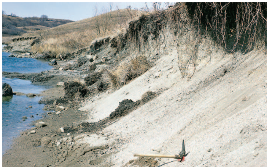
Figure 2. Erosion by groundwater sapping (one week of freeze-thaw cycles) on shoreline bank of Lake Ashtabula, North Dakota, USA. With melting of lake ice, wave action removed the talus.
