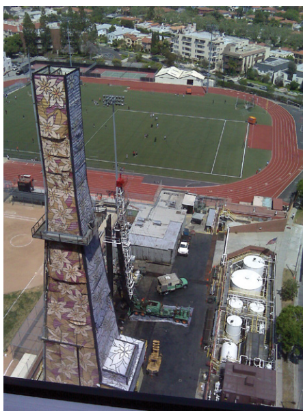
Figure 3. The “Flower Tower” used to conceal an oil rig on the Beverly Hills High School campus. The floral pattern was designed by two artists who were school alums and painted by terminally ill children who were being treated in local hospitals (Tormey and Middaugh, 2014). This photo was taken during repair of the rig, which is visible behind the Flower Tower. Both the rig and its Flower Tower camouflage were dismantled in 2020. Credit: EricF2000 via Flickr.
