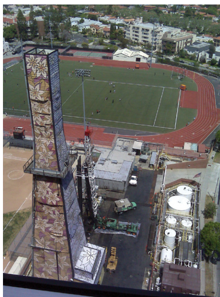
Figure 3. The “Flower Tower” used to conceal an oil rig on the Beverly Hills High School campus. The floral pattern was designed by two artists who were school alums and painted by terminally ill children who were being treated in local hospitals (Tormey and Middaugh, 2014). This photo was taken during repair of the rig, which is visible behind the Flower Tower. Both the rig and its Flower Tower camouflage were dismantled in 2020. Credit: EricF2000 via Flickr.
