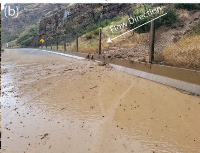
Figure 4. Differences in flow size from the first to third year after the wildfire. (A) A debris flow during the first postfire summer (2021) depositing material on both east-bound and west-bound highway lanes, as well as in the Colorado River. (B) A sediment-laden flow during the third year after the fire (2023) depositing material behind a concrete barrier with minor mud on the highway. (Photo credits: Colorado Department of Transportation).
