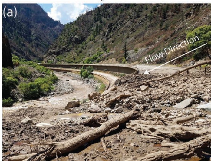
Figure 4. Differences in flow size from the first to third year after the wildfire. (A) A debris flow during the first postfire summer (2021) depositing material on both east-bound and west-bound highway lanes, as well as in the Colorado River. (B) A sediment-laden flow during the third year after the fire (2023) depositing material behind a concrete barrier with minor mud on the highway. (Photo credits: Colorado Department of Transportation).
