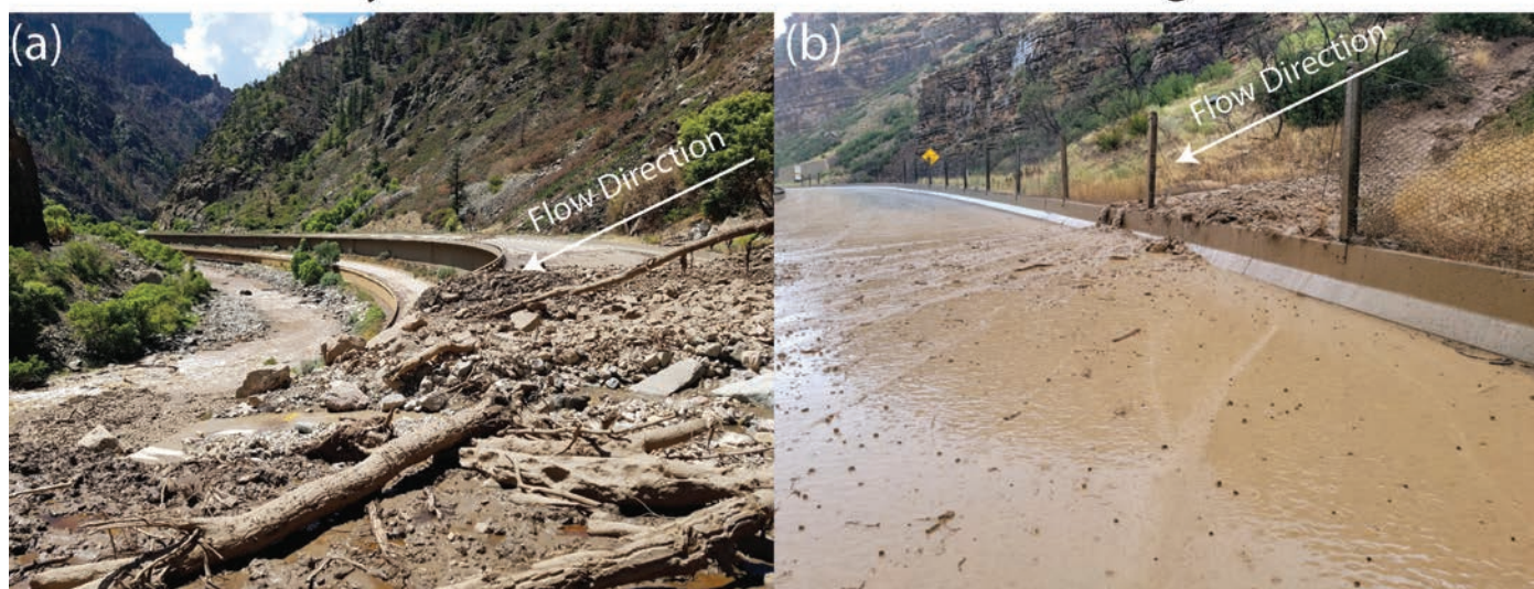
Figure 4. Differences in flow size from the first to third year after the wildfire. (A) A debris flow during the first postfire summer (2021) depositing material on both east-bound and west-bound highway lanes, as well as in the Colorado River. (B) A sediment-laden flow during the third year after the fire (2023) depositing material behind a concrete barrier with minor mud on the highway. (Photo credits: Colorado Department of Transportation).
